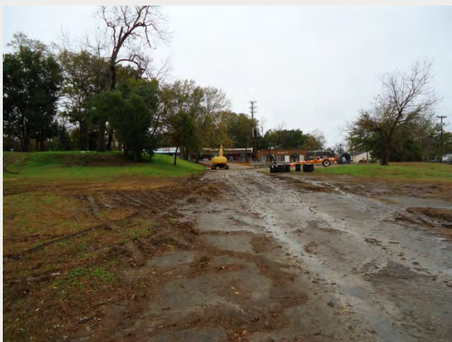
VIEW FROM SITE TO THE SOUTH
